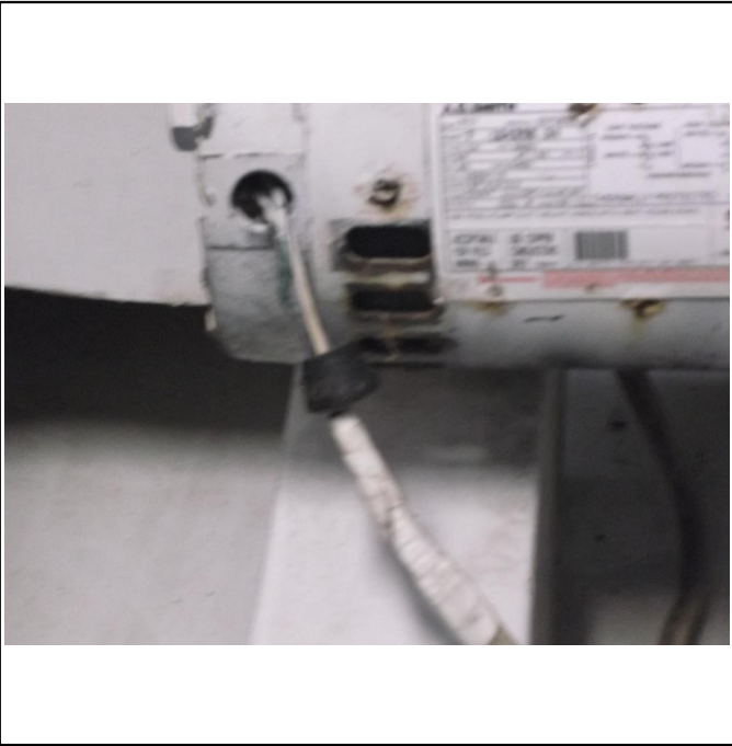
A/C Pump Wiring
