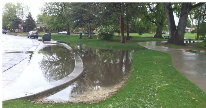
FIGURE 6. Failing stormwater system (Source: Muller Engineering. 2015.)
