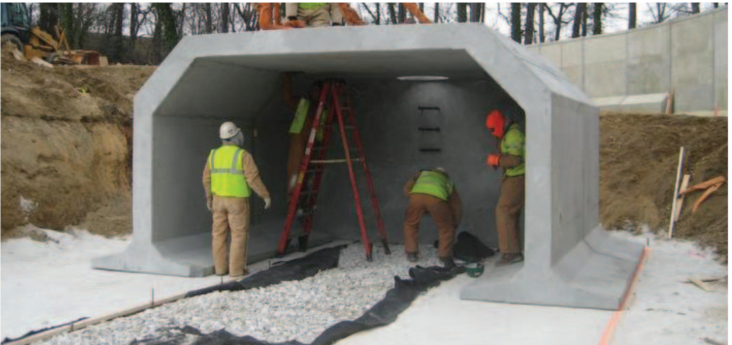
Large pre-cast concrete detention tanks being installed
