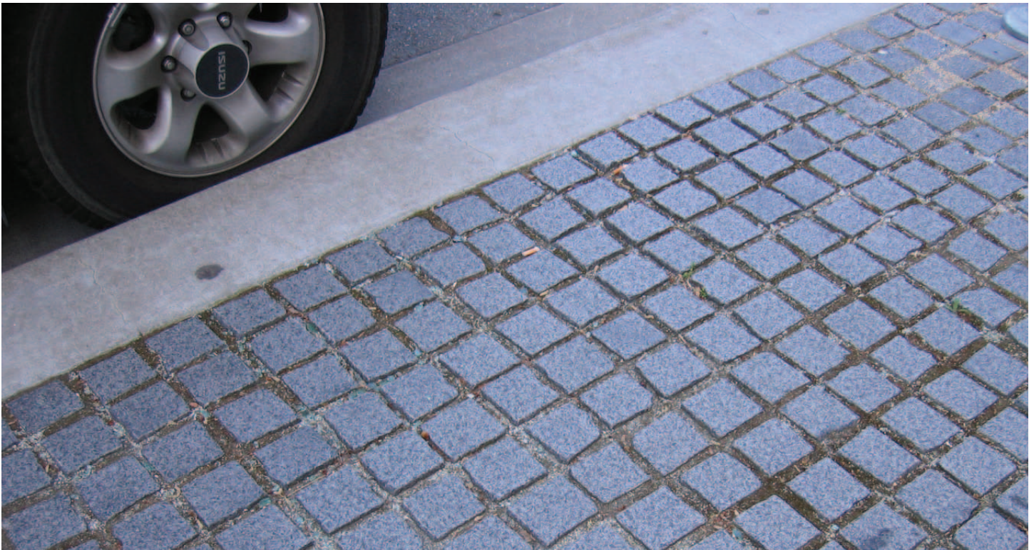
Porous paving underdrained
