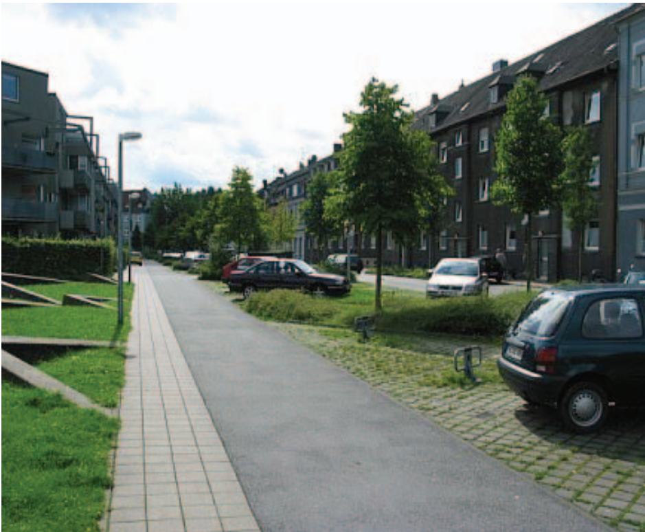
Permeable paving used for parking areas in Germany
