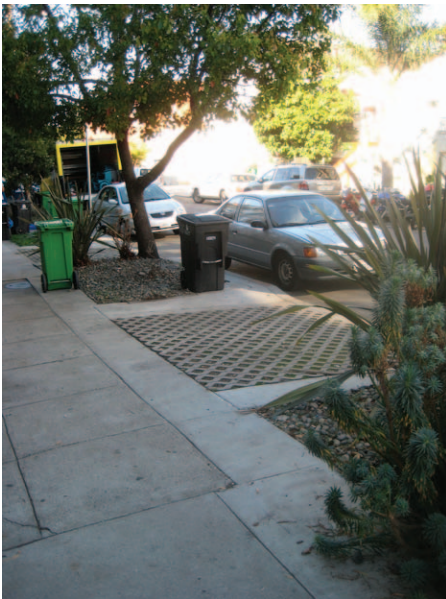
Permeable paving used for driveway aprons on Shotwell Street in San Francisco, California
