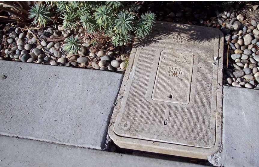
▲ Utility vaults may be located within planting areas as long as access is maintained
