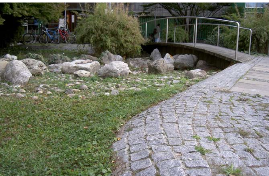
▲ Pathways across pocket parks and other large open space areas in the right-of-way can be raised to allow infiltration below Source: Sherwood Design Engineers
