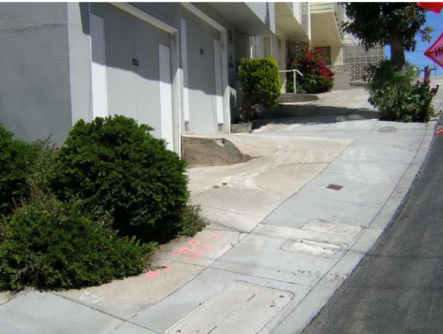
▲ Many streets have few or no trees for entire block lengths because subsurface utilities limit the ability to plant
