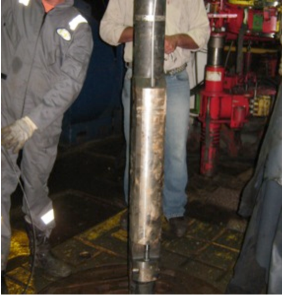
Figure 1: Installation of PCP Monitoring System
