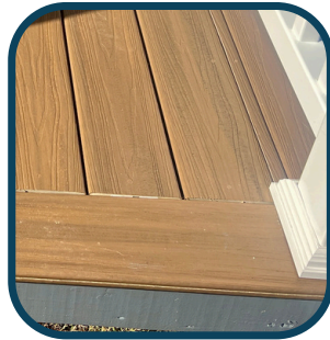
Composite Deck Porch
