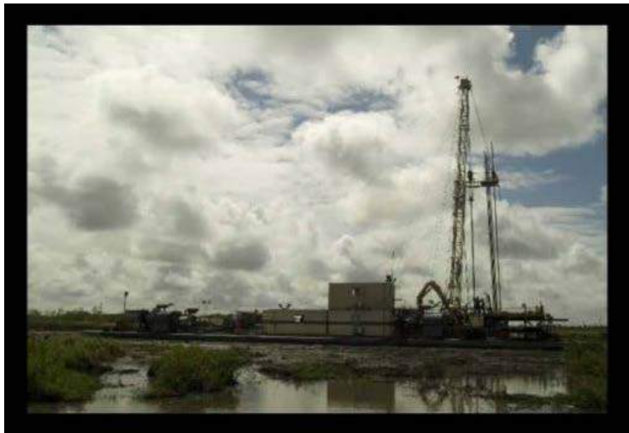
ACV production platform in operation, United World Energy Corp., Suriname (2007)
