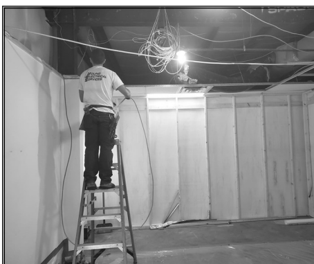
Working on the new wellness room at Riverway
