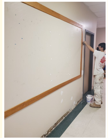
Preparing to paint the hallways at Riverway
