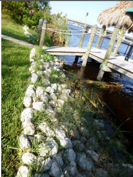
Photo 5: Additional view of unauthorized riprap along the shoreline of Property 1. Facing west.
