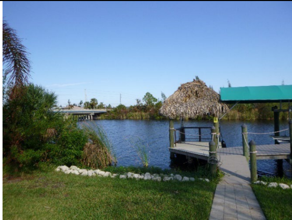
Photo 3: View of unauthorized riprap along the shoreline of Property 1. Facing north.
