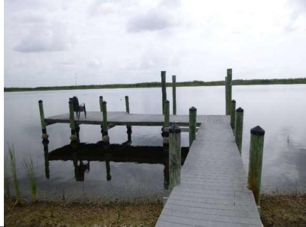
Photo 1: View of unauthorized docking structure on Property 1. Facing east
