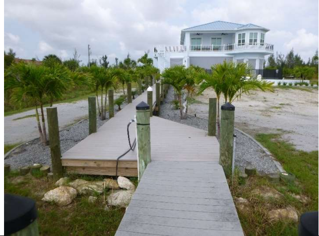
Photo 2: View of unauthorized docking structure/boardwalk in wetlands on Property 1. Facing west
