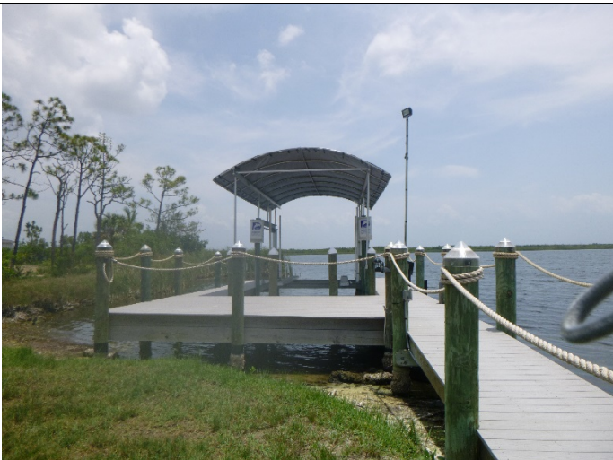
Photo 5: Facing East, view of dock and covered canopy.
