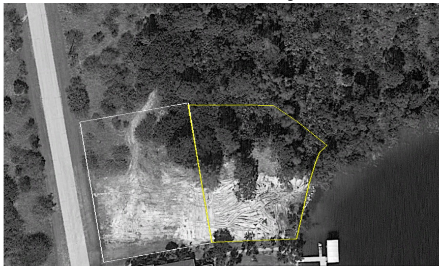
Figure 3: Aerial photograph dated 2/17/2014 showing first impacts to wetlands via clearing of vegetation. The Greenbelt section is outlined in yellow, and Property 2 is outlined in white. Source: Google Earth.
