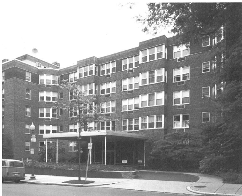
The severely plain facade of the Carlyn is slightly relieved by the horizontal bands of dark red brick that appear on the top floor.
