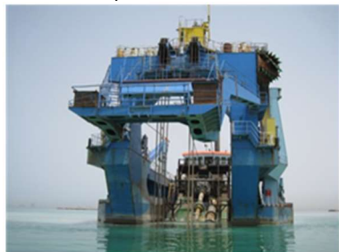
Cutter suction dredging to -9m Chart Datum
