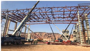
53m span steel truss (32T) & 25m concrete lift shafts
