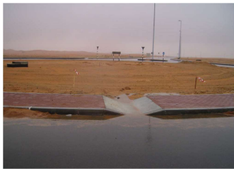
Kerb spillways to soakaways adjacent to roads
