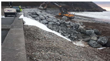
Friog: rock toe protection to existing embankment
