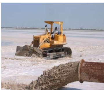
Land reclamation of pumped dredged material
