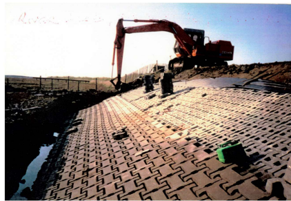
Revetment block placement on flood embankments along the River Alde in Suffolk, 1992 to 1993
