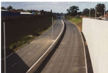
A47 bypass constructed along old rail line, comprised grade-separated junction and roundabouts, 1991
