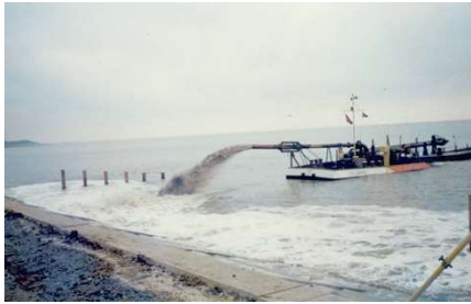
Beach recharge with similar beach grading mix using trailer suction hopper dredger, 1988 to 1990
