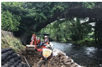
Bontnewydd: erosion protection to existing river wall
