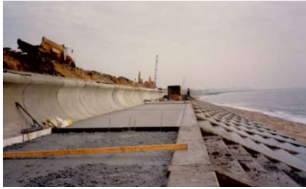
New promenade and stepped revetment at The Dip, Felixstowe, 1988 to 1990
