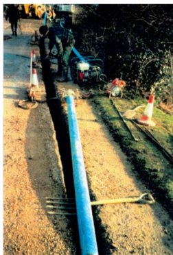
Anglian Water's programme for replacing old cast-iron mains with MDPE pipework
