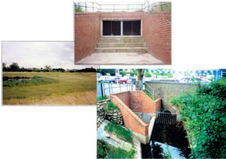
Side weir conveys storm flows along bypass to storage reservoir formed by earth embankments
