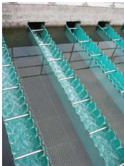
New lamella settlement (multiflo®) troughs at a water treatment facility in China
