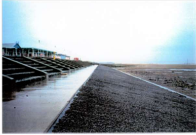
Additional open-stone asphalt apron and toe cut-off to existing defences at Y Ffrith Beach, Prestatyn
