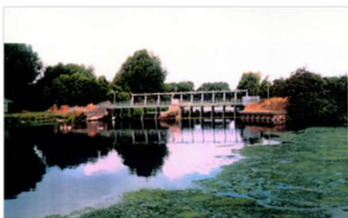
Vertical gates at Kings Weir, Oxford required replacement with radial gates
