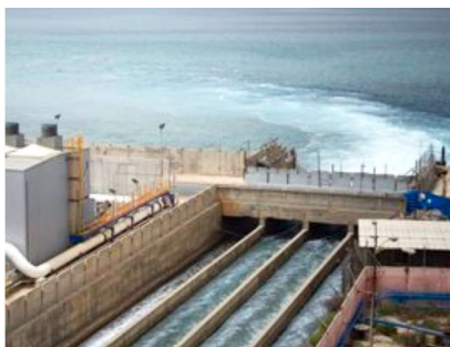
Simulation of flushing in the Red Sea indicated that intake point and outlet canal (via DRI steel plant) at the KAEC desalination plant to be 300m apart
