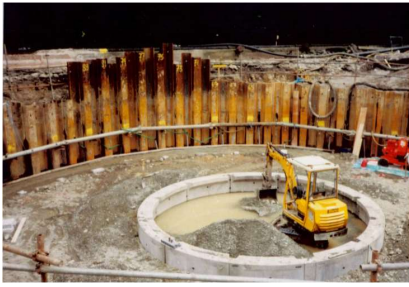
Precast concrete segments to form central hopper of a new settlement tank
