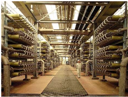
Membrane (Ultra-filtration, Reverse Osmosis) Systems for De-Mineralized Water & Industrial Water
