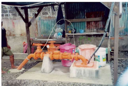
Typical groundwater well encountered in Philippines, and poor condition of chlorination equipment
