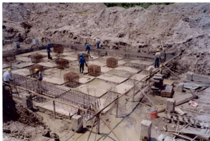
Construction of pile cap and base slab for rapid gravity sand filter unit at Fort Bonifacio, Manila, 1998
