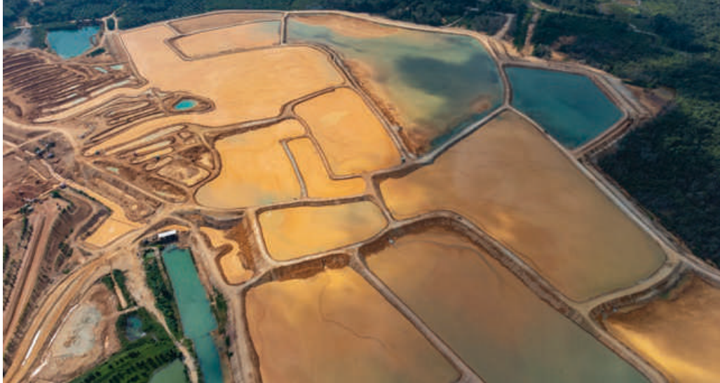
Pengelolaan Residu Bauksit di CITA Bauxite Residue Management at CITA
