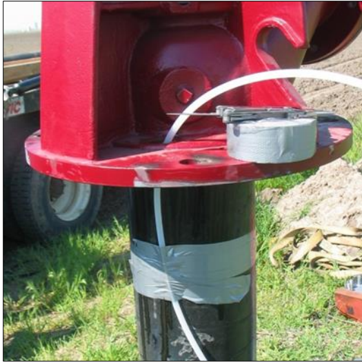
Fig. 8. The air line is secured to the column pipe with a final wrap of duct tape. The tubing is run through the bottom end of the pump stand access hole. (NOTE: Both figs 7 and 8 show duct tape being used to secure the tubing to the column pipe. Current recommendations are to use plastic zip ties or large hose clamps instead).
