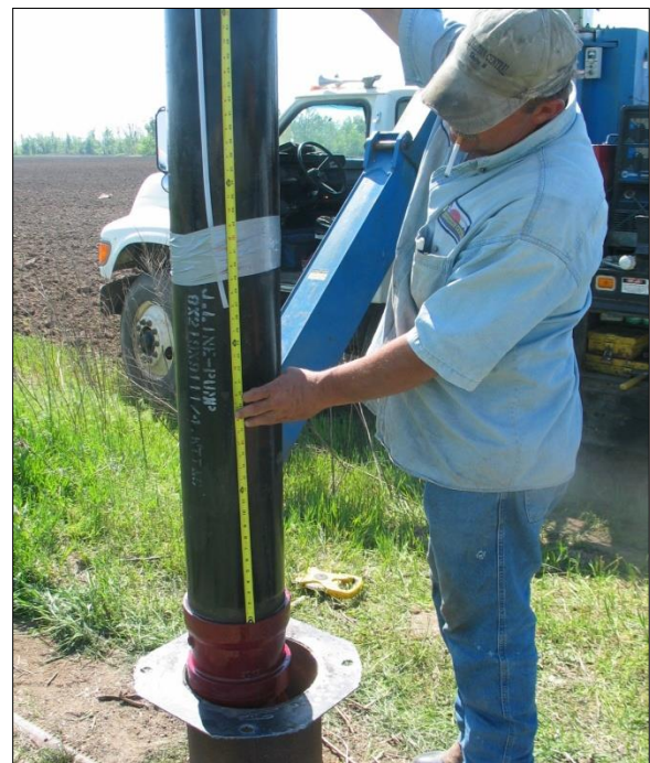
Fig. 7. The distance from the end of the tubing to the top of the pump being measured. Make sure that the end of the tubing is at least 2 feet from intake of the pump.
