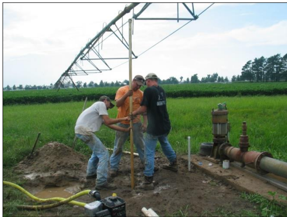
Fig. 4. A monitor well being installed near an irrigation well which lacks enough space between well casing and column pipe for an air line.
