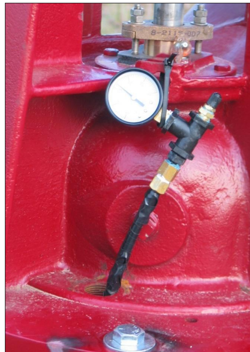
Fig. 9. The air gauge unit attached to pump stand with a zip tie and exposed tubing wrapped with electrical tape to shield the tubing from the sun's UV light.
