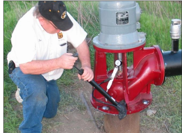
Fig. 11. Using a bicycle pump to air up an air line.
