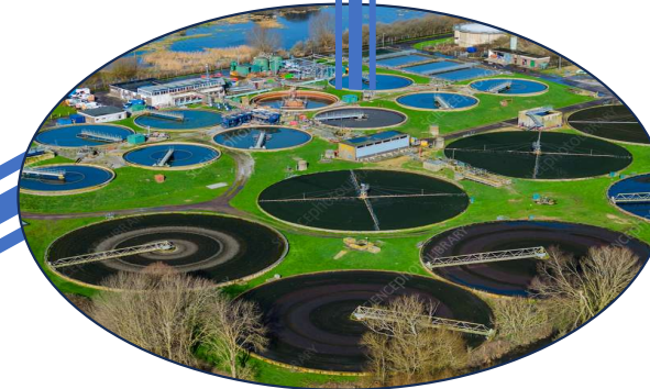
Waste-Water Treatment Plant
