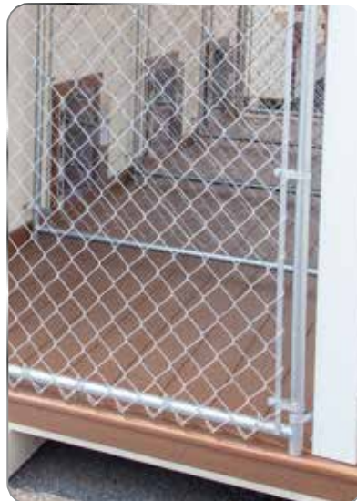
COMPOSITE DECKING ON RUNS
