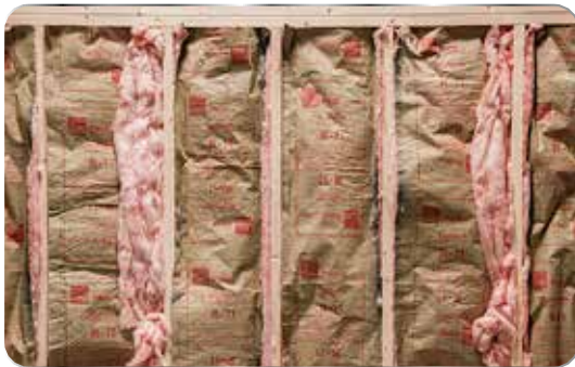
R-13 Batten Insulation In Walls & Ceiling
