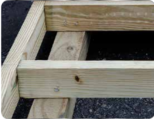
Pressure Treated 2x4 Floor Joists 4x6 Runners
