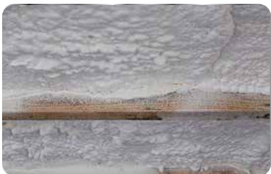
R-13 Closed Cell Spray Foam Insulation in Floor
