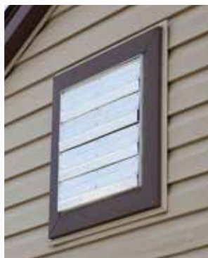
16" 110-V Exhaust Fan w/Aluminum Gable Shutters 1900 CFM 1.35 AMPs
