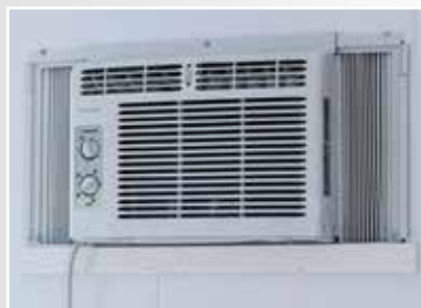
A/C Unit Installed
