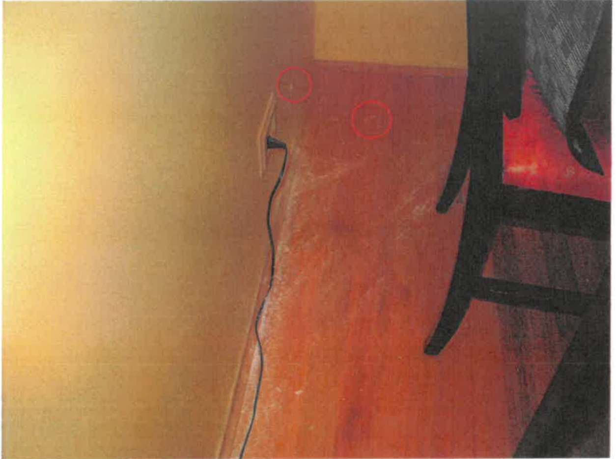
Exhibit 4 – IMG_2223.jpg: Dining room walls and floor
