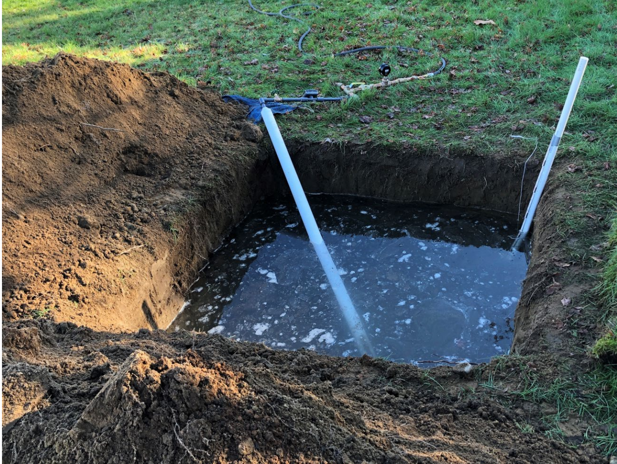
Fig. 1: Photograph of an infiltration test in an excavated pit.
