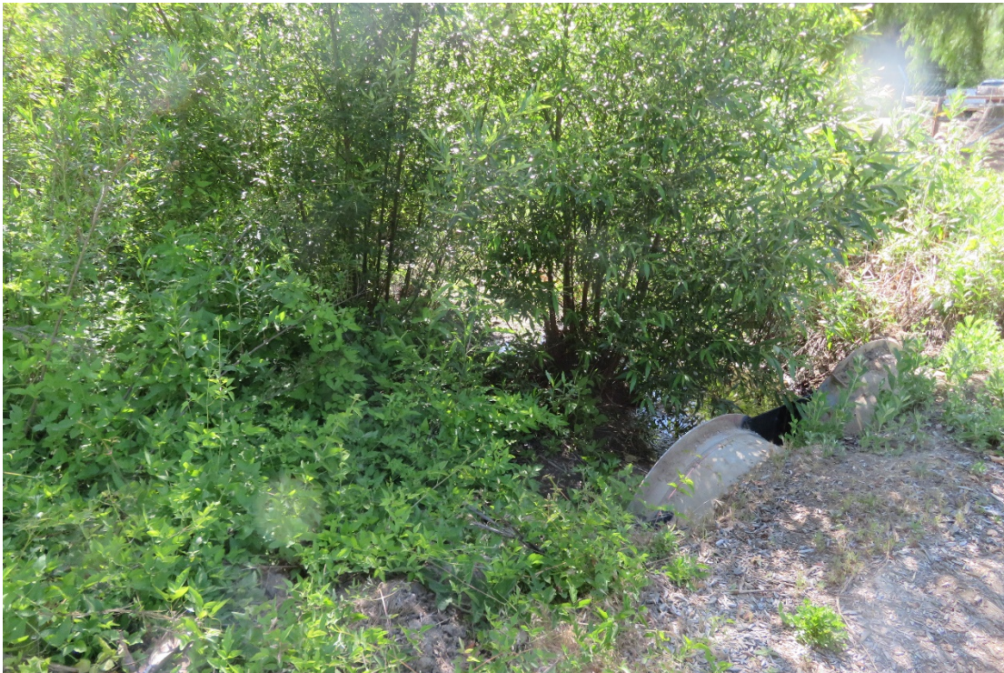
Clear the brush in the discharge channel of the auxiliary spillway
