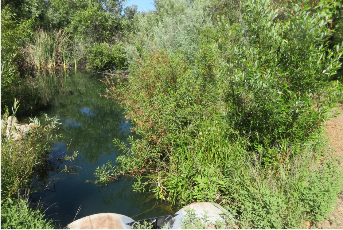
Clear the brush along both sides of the approach channel to the auxiliary spillway
