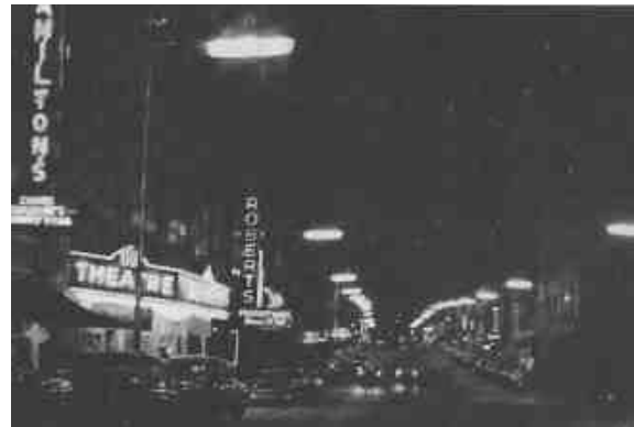
The new four lane highway gave a new look to downtown Harriman, especially with new night lighting
