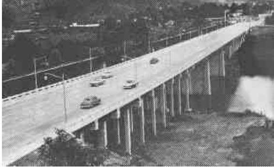
William Hamilton Browder Bridge (Hwy 27) became the progressive access point to downtown Harriman in 1957
