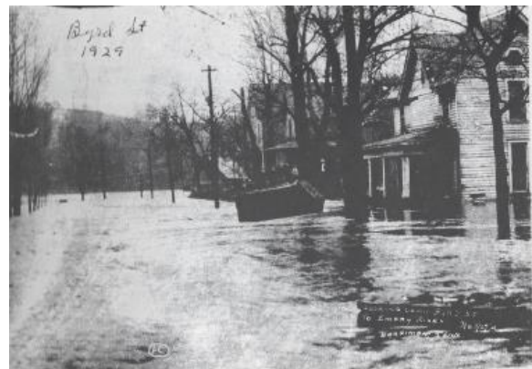
Flood photos taken by C. W. Adkisson, Sr. in this Newsletter are part of a photo album in Walter Pulliam’s Harriman: The Town That Temperance Built
