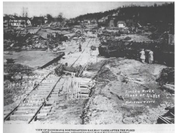
VIEW OF HARRIMAN & NORTHEASTERN RAILWAY YARDS AFTER THE FLOOD NOTE: Overturned cars, collapsed American Park & Hoe Company's Building
