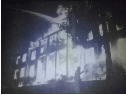
The Mossop School Building Fire in the 1980s
