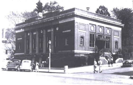
Still a prominent building in downtown, the post office was the center of business and social life in Harriman until 1980
