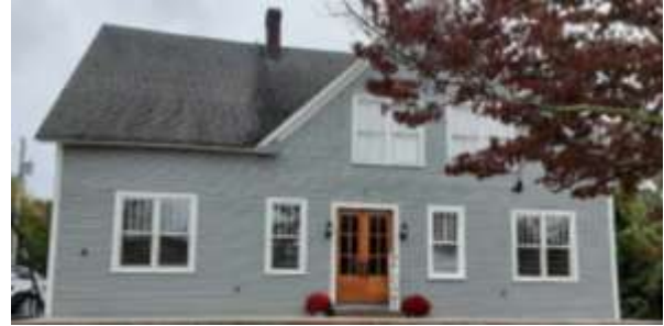
These windows are actually a combination of “old wood” and replacements that are manufactured to match the style
