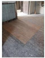
patch (pun intended) addressed constraint moving forward with sanding the floors. Pat worked during the week to salvage floor boards from the Sanctuary altar and (stage) area, reuse them as
