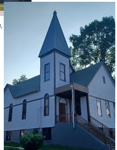
Harriman Hall Renovations, June 2023
