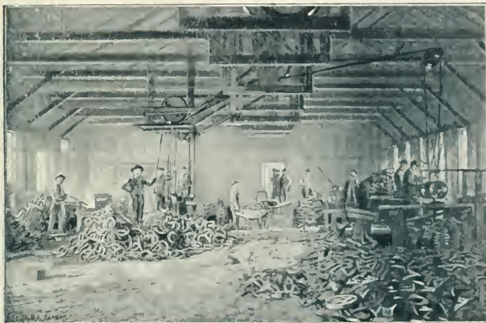
FORGE ROOMS, AGRICULTURAL WORKS.
