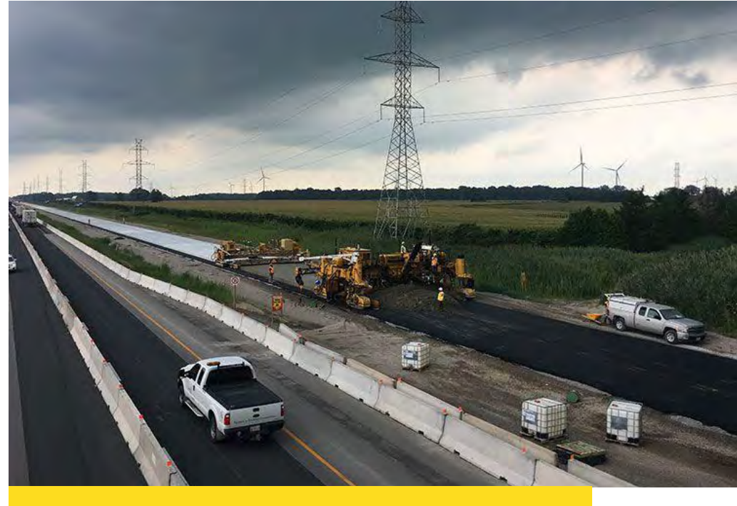
Highway 401 Widening, ON Canada
