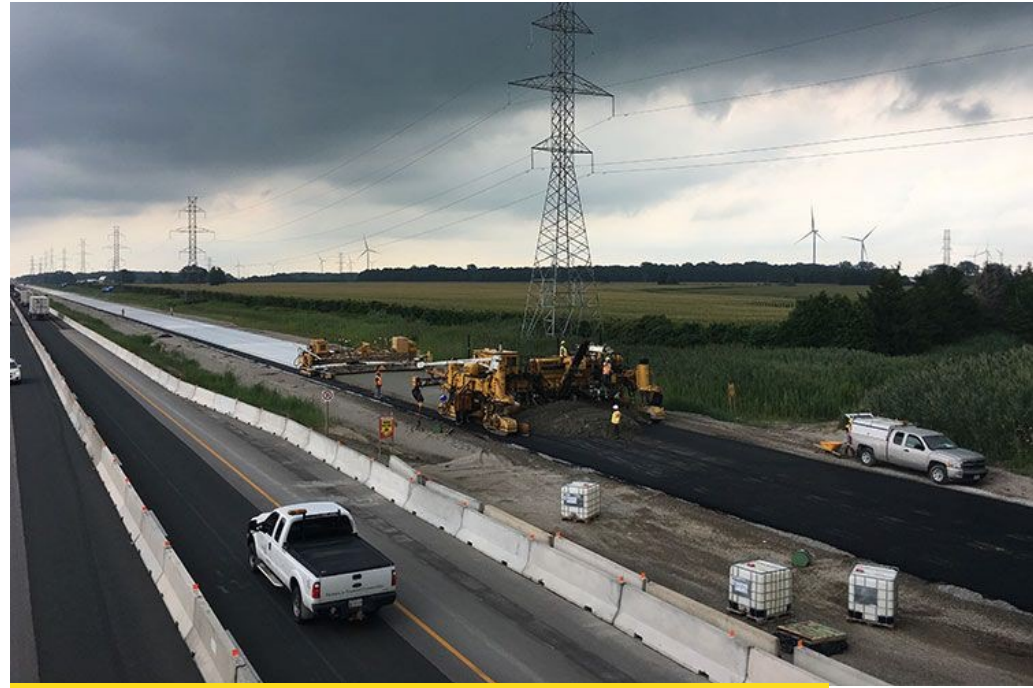
Highway 401 Widening, ON Canada
