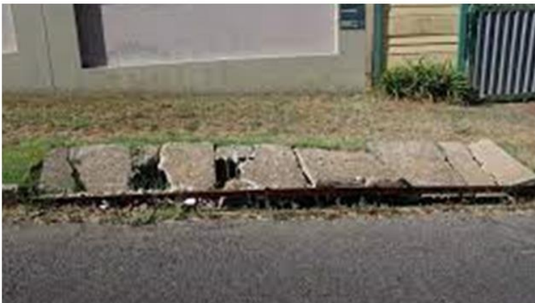
DISLODGED / BROKEN KERB INLET (KI) on Storm water drains
