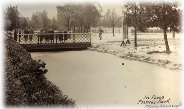
Princes Park: Main Drain in flood circa early 20 th Century.
