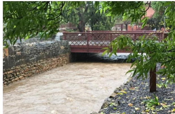
The same location more than 120 years later following the heavy rain in mid- October this year.
