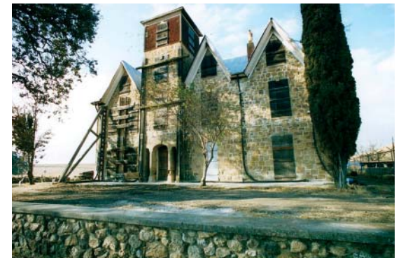
The restoration of the Marsh House
