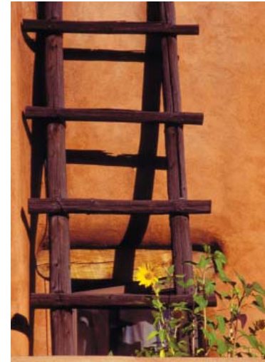
Historic adobe structure
