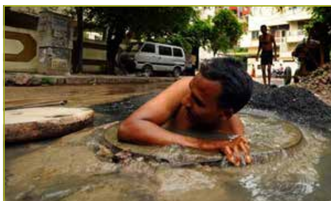
Figure 69: A sewerage worker clears a choked drain
