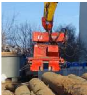
7PHFV Vibro Installing an 800 m Long Sheet Pile Wall To Reinforce The Loire River Banks.
