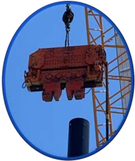
PTC 75 Driving Pipe Pile at the LCRA Pump Station in Bay City, TX
