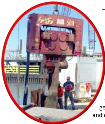
HPSI Model 500 Vibro in New Orleans, LA
