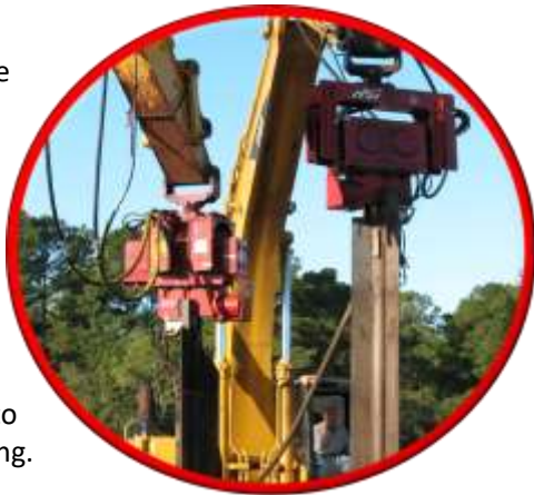
HPSI Model 100 Vibro in Galveston, Texas
