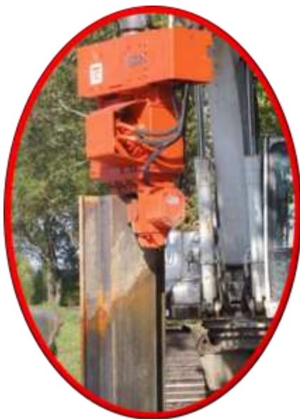
7PHFV Vibro Installing an 800 m Long Sheet Pile Wall To Reinforce The Loire River Banks.
