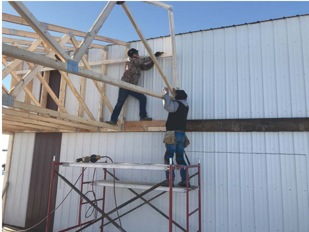
Trig Clark and Brian Flatmoe connecting the rafters to the existing building.
