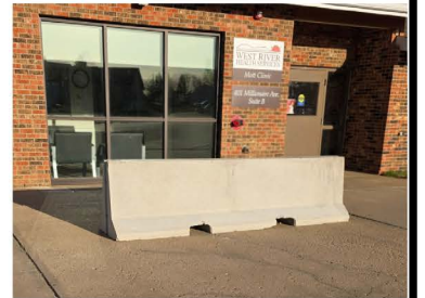
Blockade to be replaced with columns
