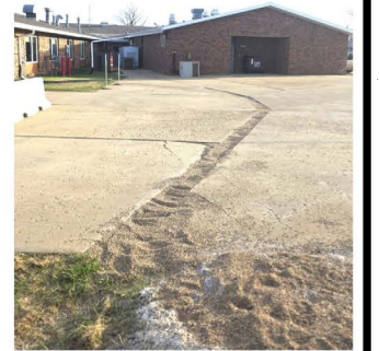
Current parking lot drainage
