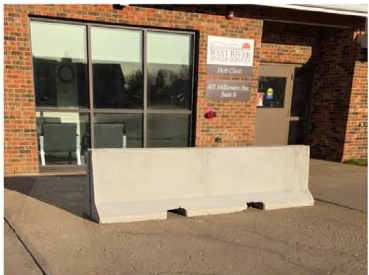
Blockade to be replaced with columns
