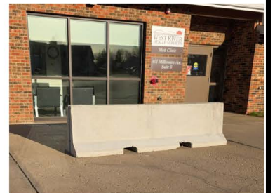
Blockade to be replaced with columns
