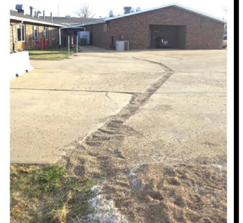
Current parking lot drainage
