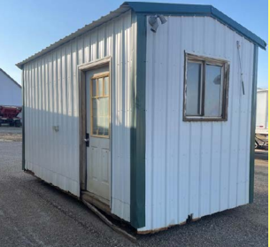
Electrical Building - 8' x 16' - Lemmon - Brannon Peterson - 605-645-1060
