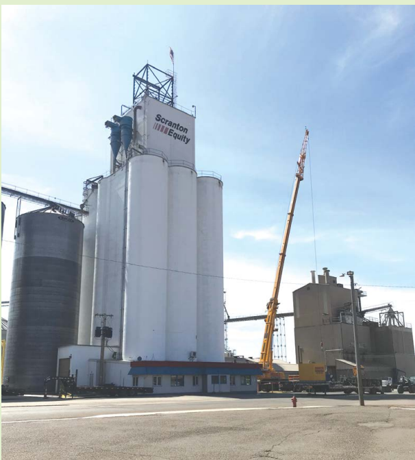
Crew working on repairs at the Scranton Equity Elevator
