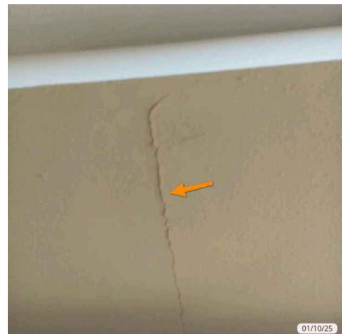
Office. Room addition
