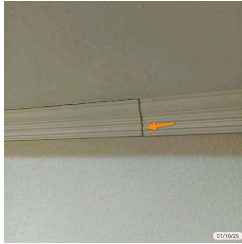
Office. Room addition
