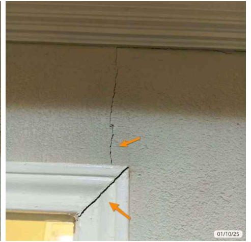
Office. Room addition
