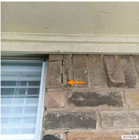
Left exterior. Soldier bricks
