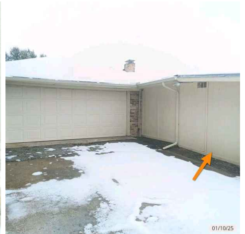
Floating patio. Attached storage closet
