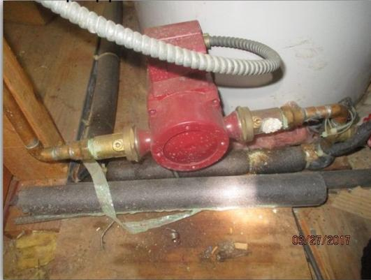
Deterioration of drain lines. No active leaks found.
