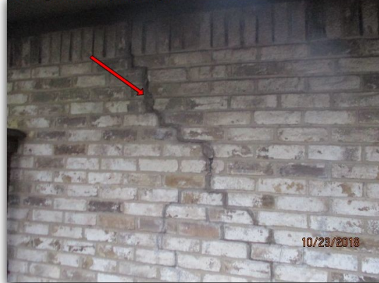
Cracking around property.
