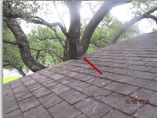
Tree in contact with roof at front.
