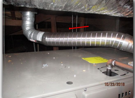
Left zone exhaust run downhill.
