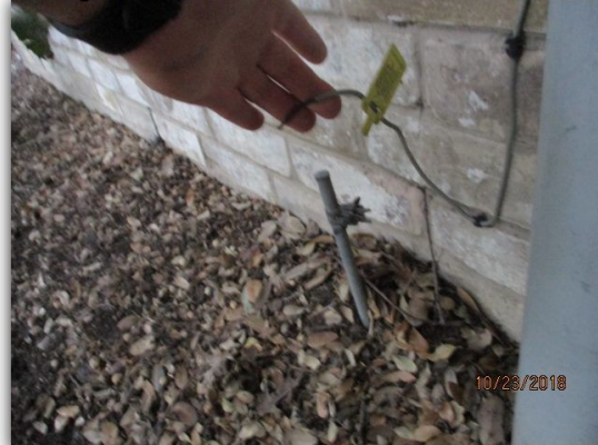
Exterior ground wire not connected.
