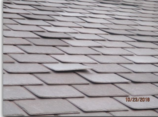
Unusual warping, lifting of material.
