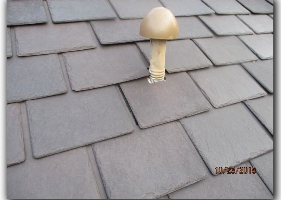
Improper installation at flashings.
