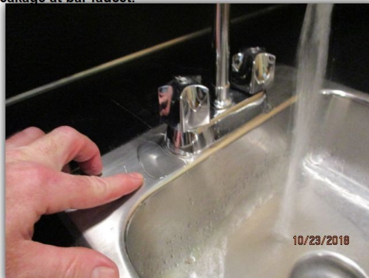
Leakage at bar faucet.
