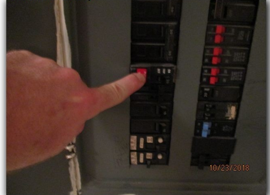
GFCI breaker not trip.
