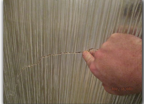
Interior drywall cracking.
