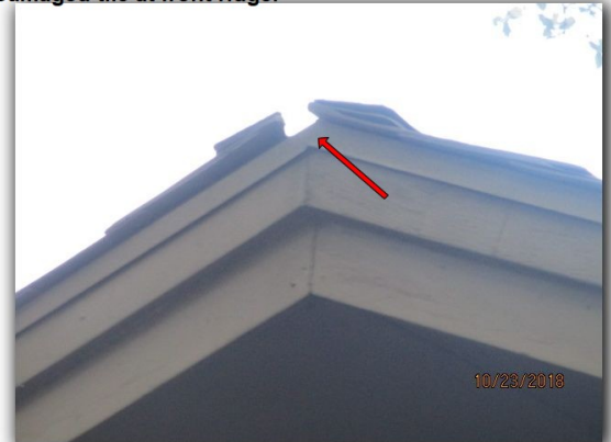
Damaged tile at front ridge.
