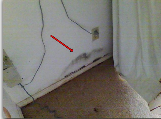
Infrared - moisture at master bed wall.
