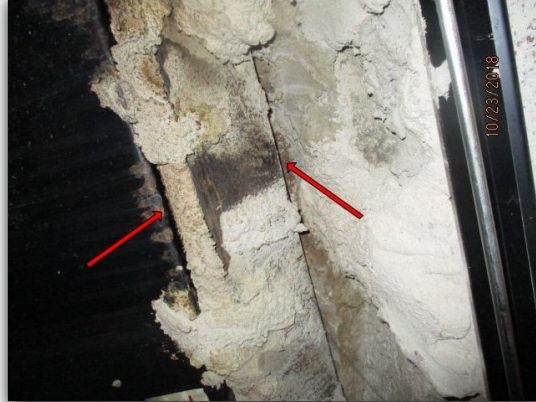
Gap at brick lintel.
