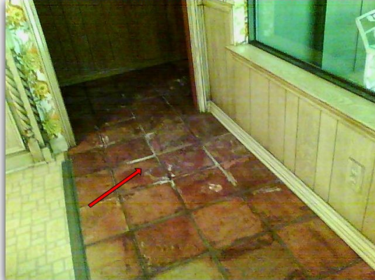
Infrared- Efflorescence. Evidence of active moisture.
