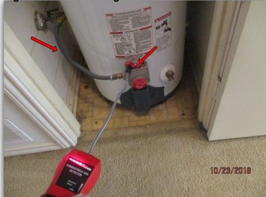
Old gas line. Gas leakage detected.
