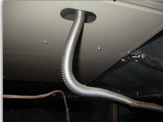
Older unit. Master zone. Gas line through cabinet.
