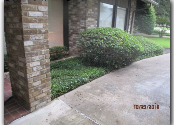
Negative slope, ponding areas.
