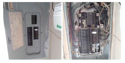
Panel Amperage(s): 200 Amp Service Electrical Panel Manufacture(s): GE
