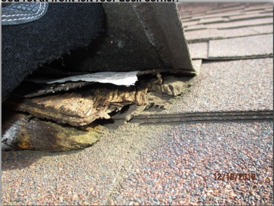
Wood rot at front left roof deck corner.
