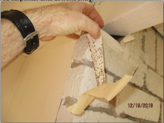
Wood rot at front left roof deck corner.
