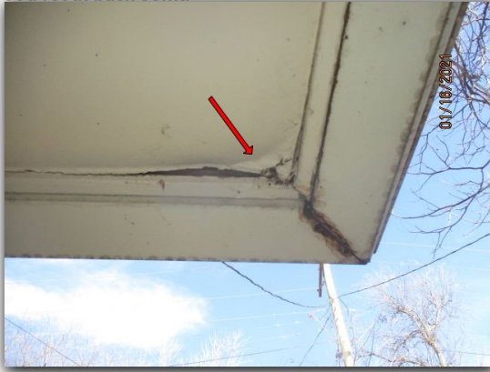
Wood rot at back soffit.
